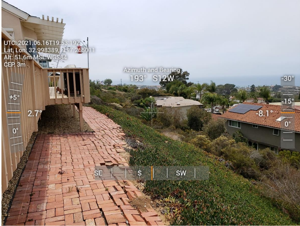
Photograph 5. Rear of residence showing iceplant-covered slope.
