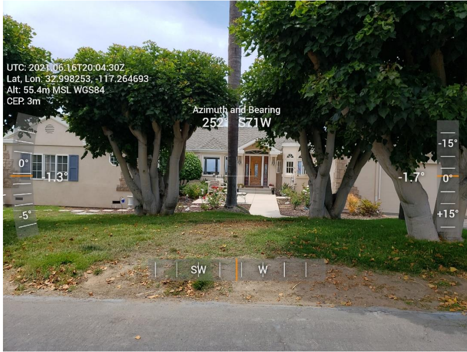
Photograph 1. View of the front of the existing residence, facing Marview Drive.
