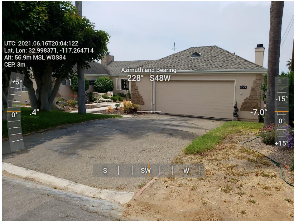
Photograph 2. View of northeast corner of the existing residence.
